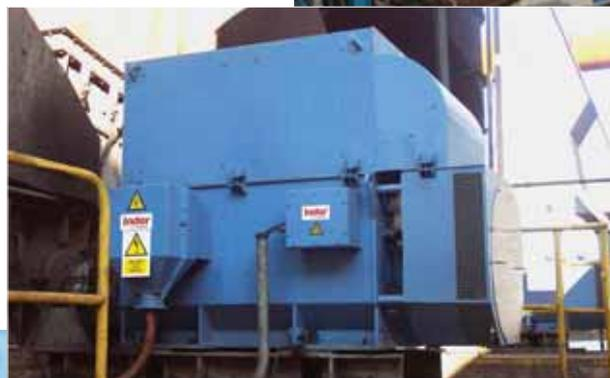
Tension reel motor in lamination plant
