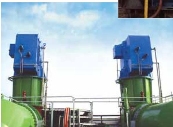
Fan drive motor in thermal plant
